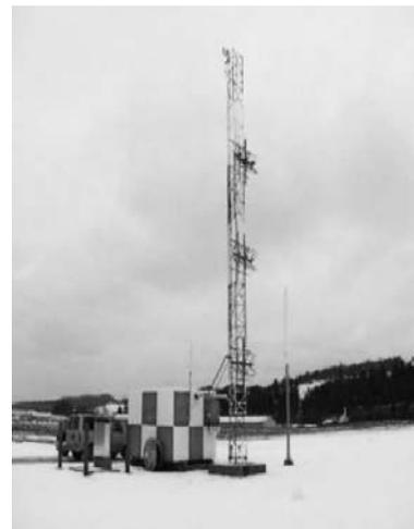
Fig. 2. Glide Slope Antenna
