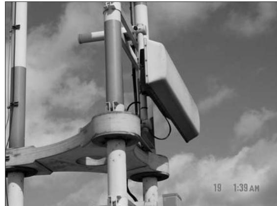
Figure 11: Antenna mast GP26. Mast joining elements are partially conductive and may have a high dielectricity constant
