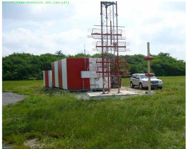
Figure 3. Picture Showing the Glide Slope Antennas Used to Generate the Proper Glide Path Angle.
