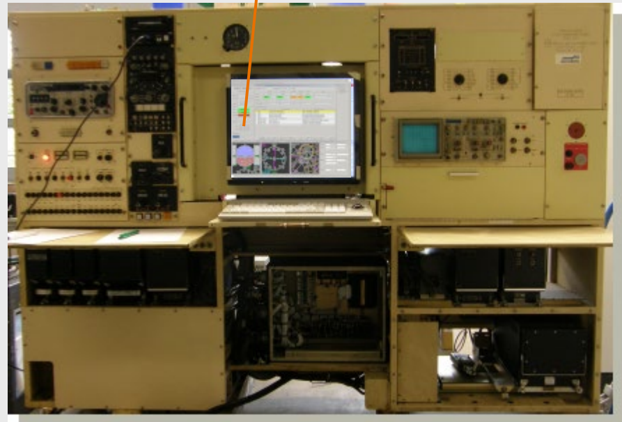
Upgraded System based on AeroFIS Technology
