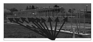
Figure 18. The Course Antenna Comprised of 16 Slotted Cable Sections
