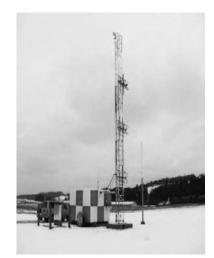
Fig. 2. Glide Slope Antenna
