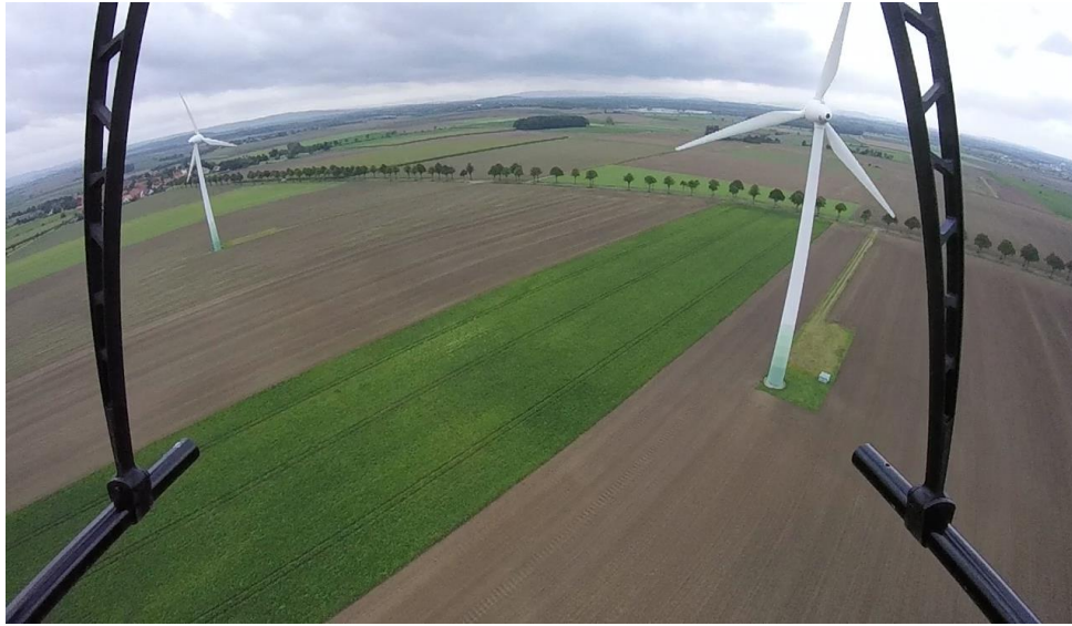
Figure 17: Flight pattern along wind turbines
