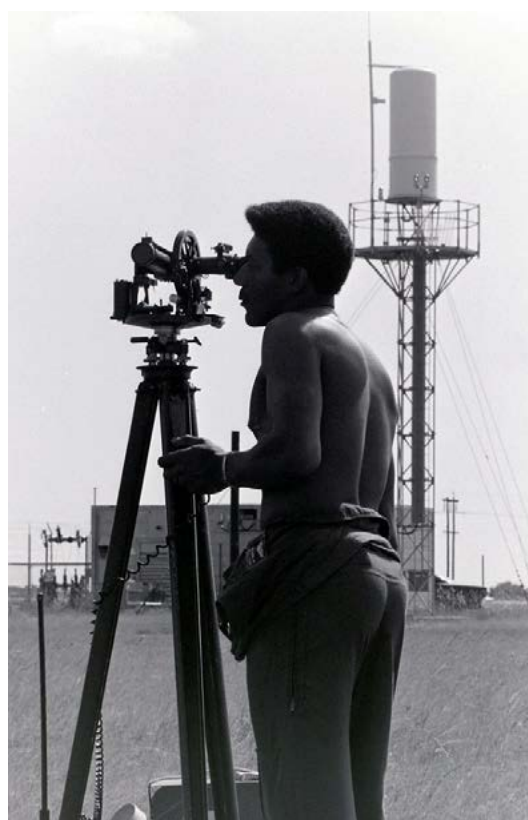
Figure 22. 1974 - USAF Theodolite operator during TACAN flight inspection at Bergstrom AFB (from USAF Flight Check Facebook Page collection)
