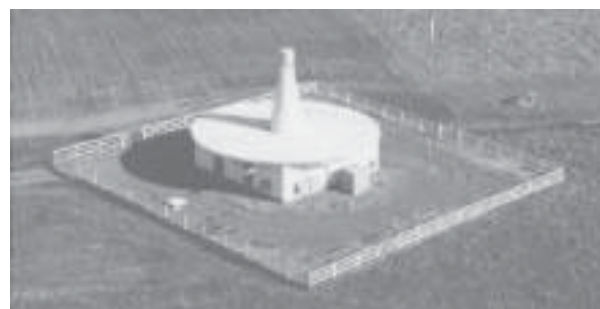
Figure 7. Circa 1950 – Early VOR ground equipment installation (from FAA archives)
