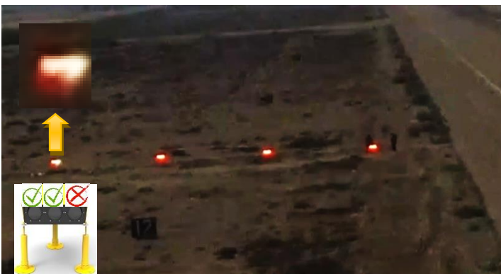
Figure 8. PAPI A Light Error
