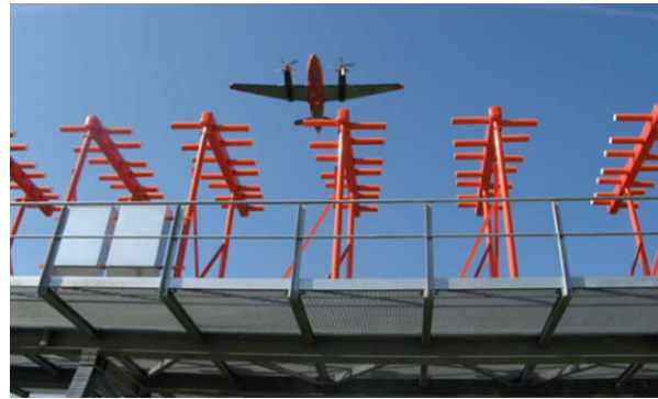
Figure 46: LSGG 04 LOC flight check
