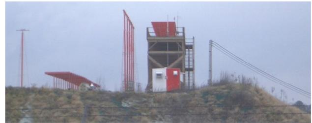
**Figure 16. Platform-Mounted CAT III Localizer.**
