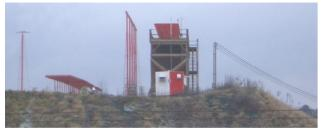
Figure 16. Platform-Mounted CAT III Localizer.
