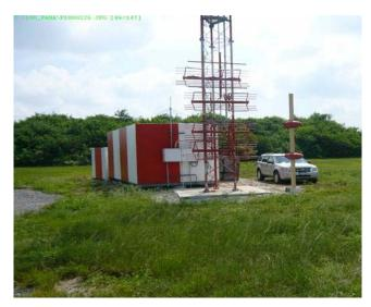
Figure 3. Picture Showing the Glide Slope Antennas Used to Generate the Proper Glide Path Angle.
