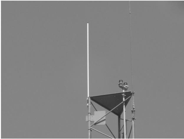
**Figure 15. Dial-up Radio Antenna**
