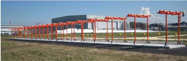
**Figure 12: Reduced Coverage Localizer Installation at Zurich Airport Runway 16**
